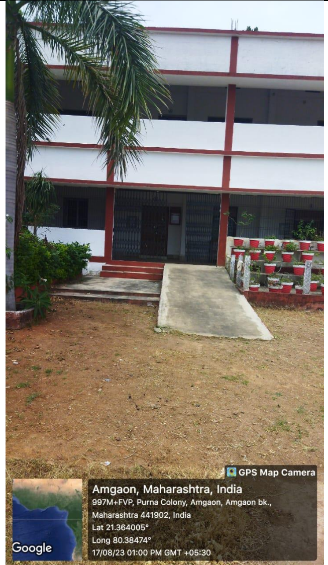
Ramp for disabled Students
