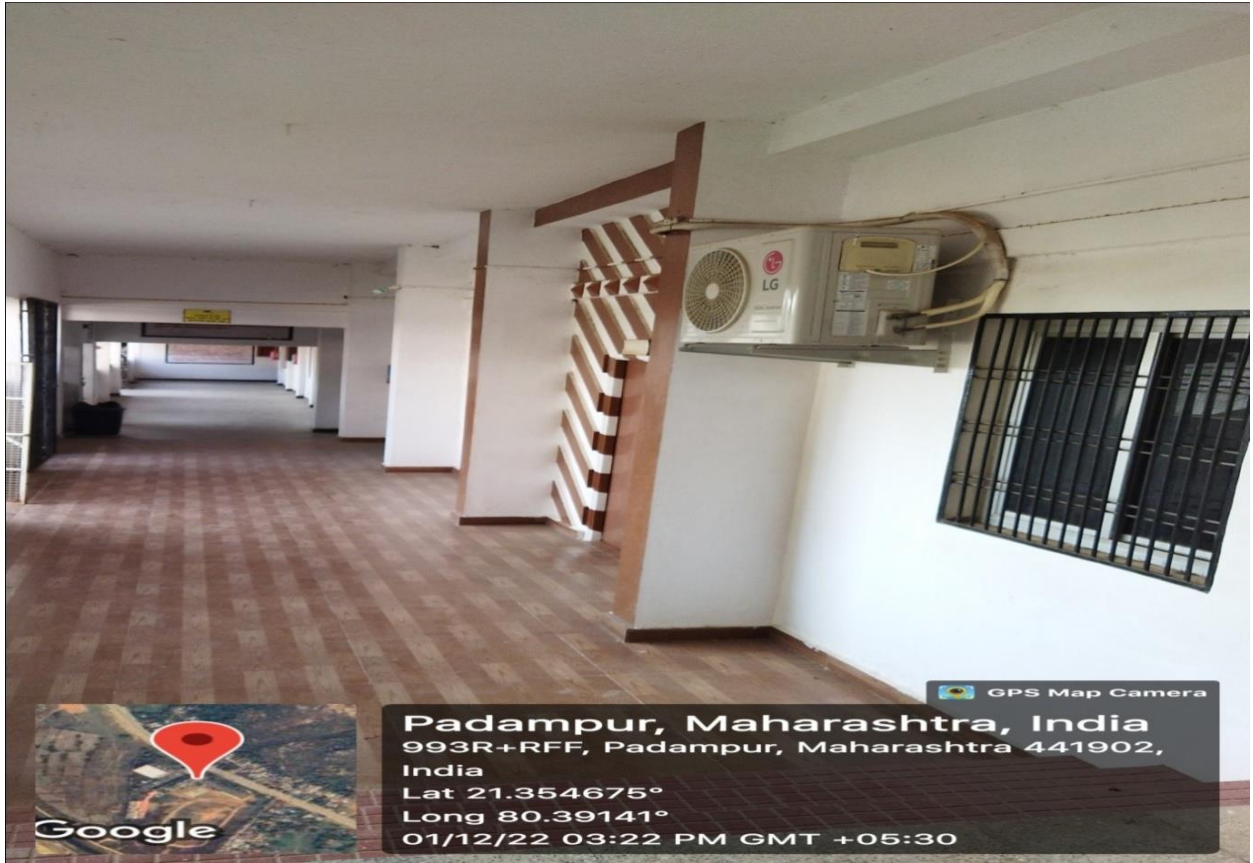
Air conditioner Installation
